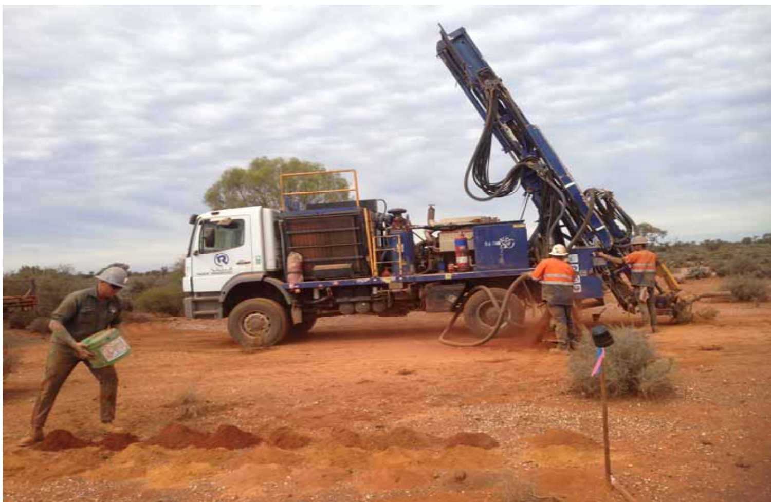
Aircore Drill Rig in Operation – Holey Dam Project
